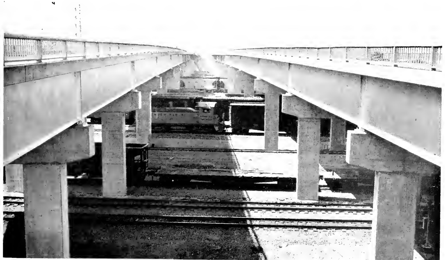
Union Pacific Railroad tracks under East Yard Overhead as viewed from the north abutment of this bridge
